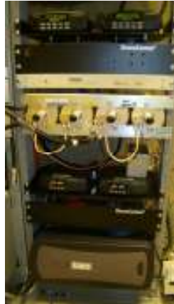
Pic of 442.275 and 224.280 repeaters & IRLP node PC
