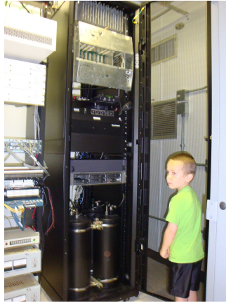
Kolton Adkins @ 145.270 site rebuild
